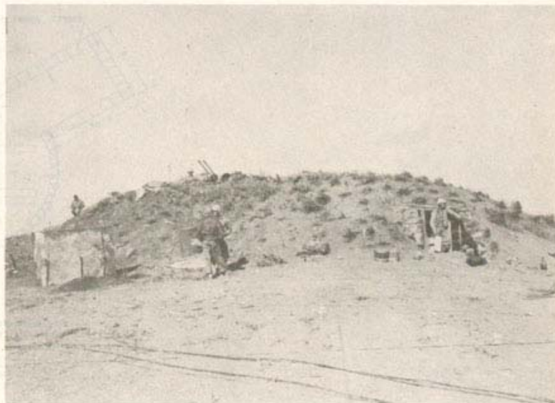
General view of earth-covered structure containing 25 mm twin-mount automatic AA position, living quarters for personnel and ammunition storage. Note the natural grass for camouflage. (TA-164E)
