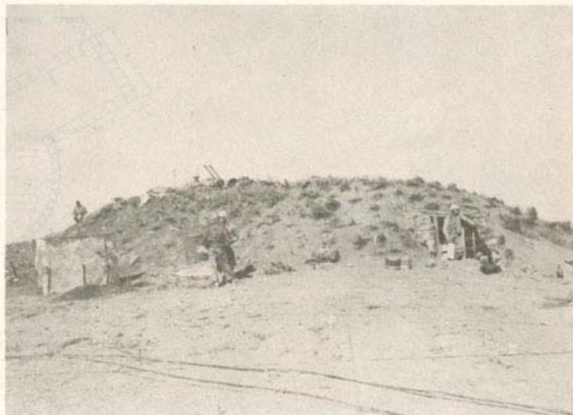
General view of earth-covered structure containing 25 mm twin-mount automatic AA position, living quarters for personnel and ammunition storage. Note the natural grass for camouflage. (TA-164E)
