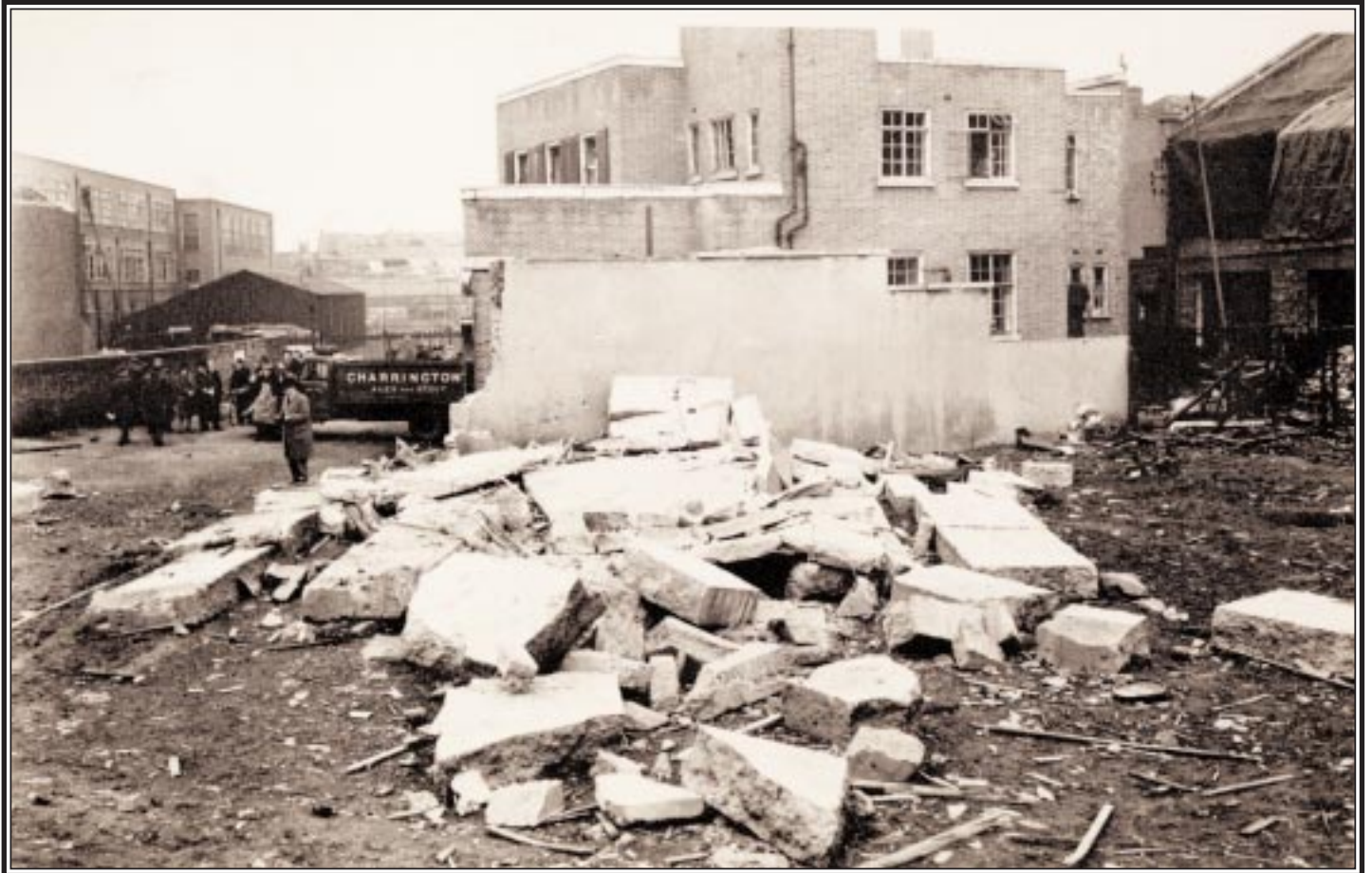
Photograph showing public shelter having been hit by a bomb
